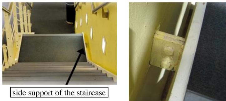
Figure 2. Detail of the side support of the staircase
